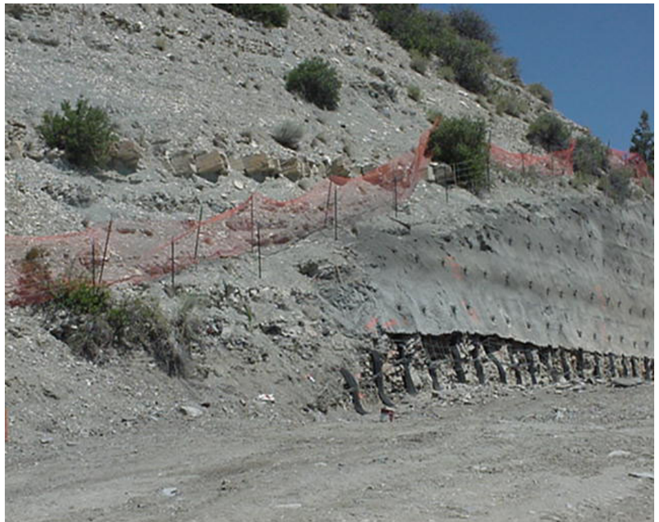
Figure 1. This talus slope is home to the Clay phacelia. The wall was constructed to prevent impacts to the plant.
